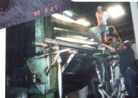
Yankee Dryer / Onsite Grinding
